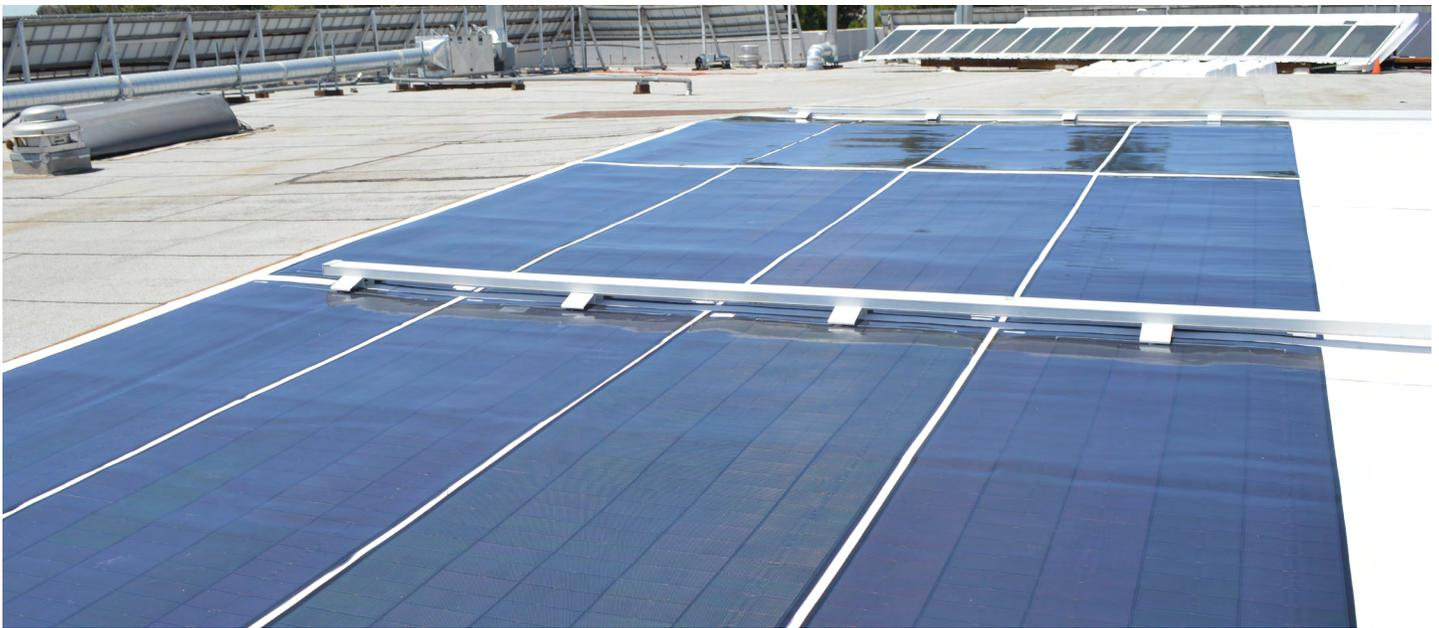
Dow's FlexsoLyt™ technology is an innovative flexible, lightweight solar module, easily installed with a peel-and-stick application and specifically designed to enable solar in your most challenging mobile and commercial structures.
